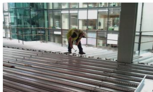
Fig. 2 Composite deck slab
